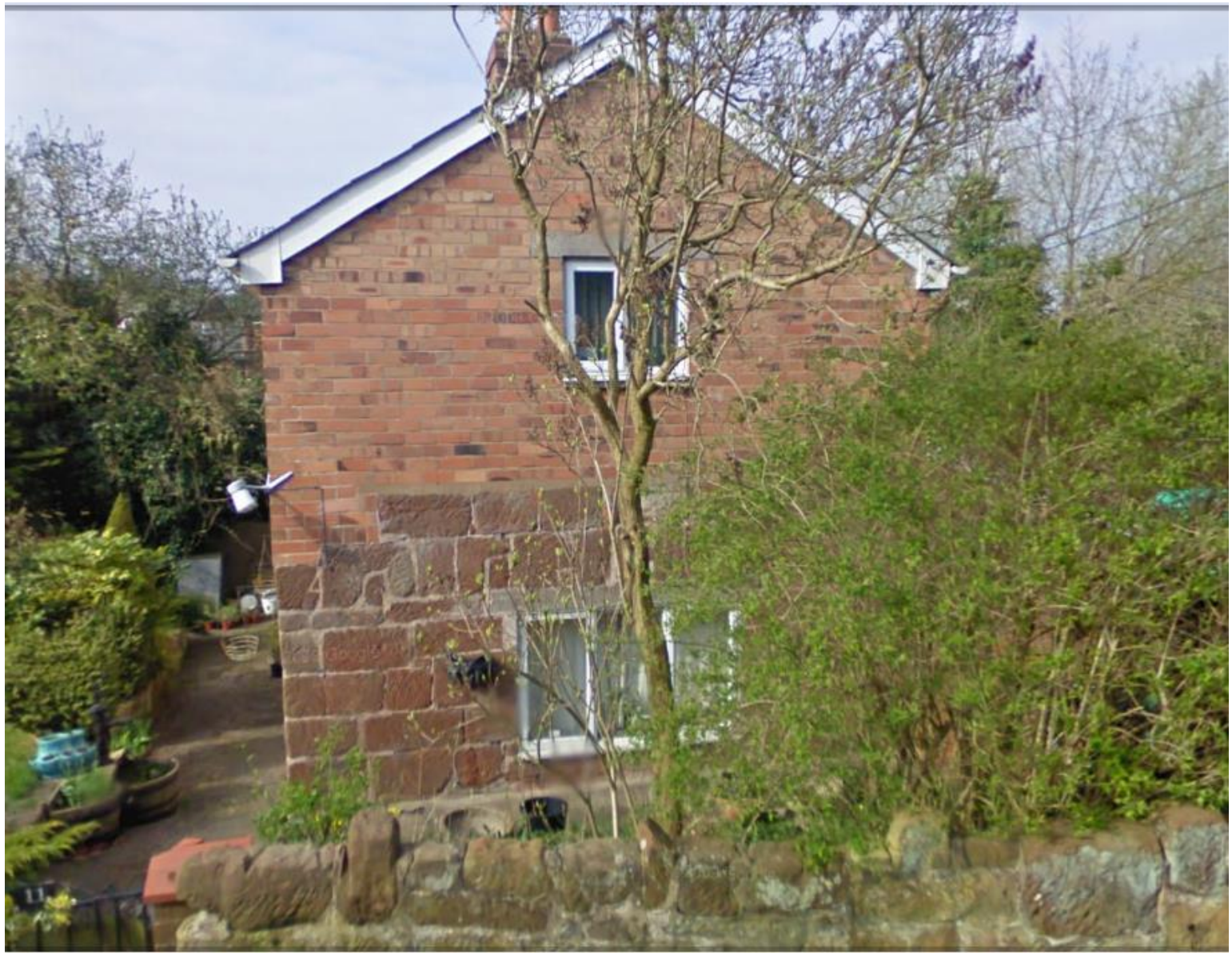
Some of the old cottages show signs of additions as in No.11 Brookside where a second story has been added.
