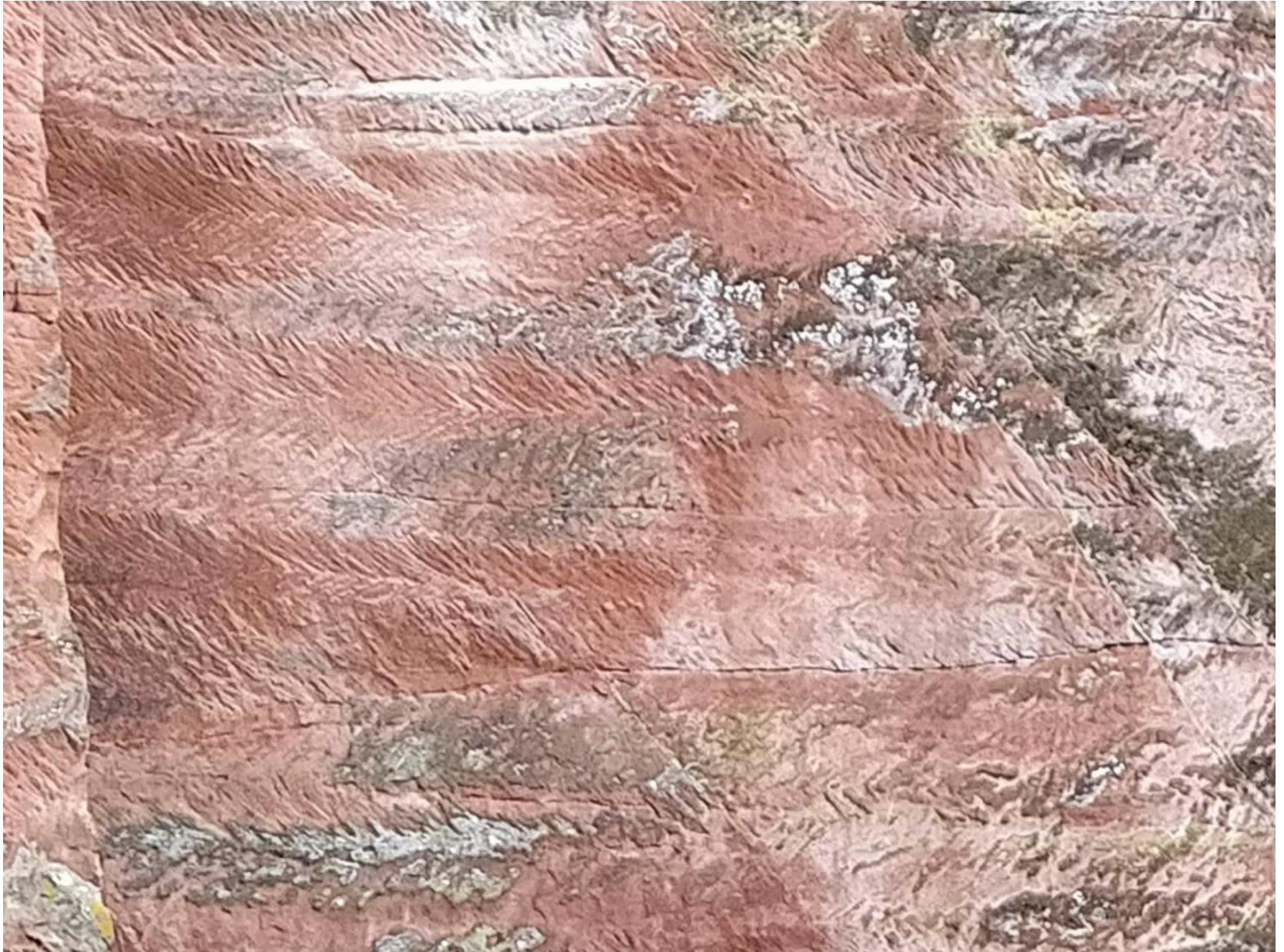
Close up of the pick strikes on the quarry walls
