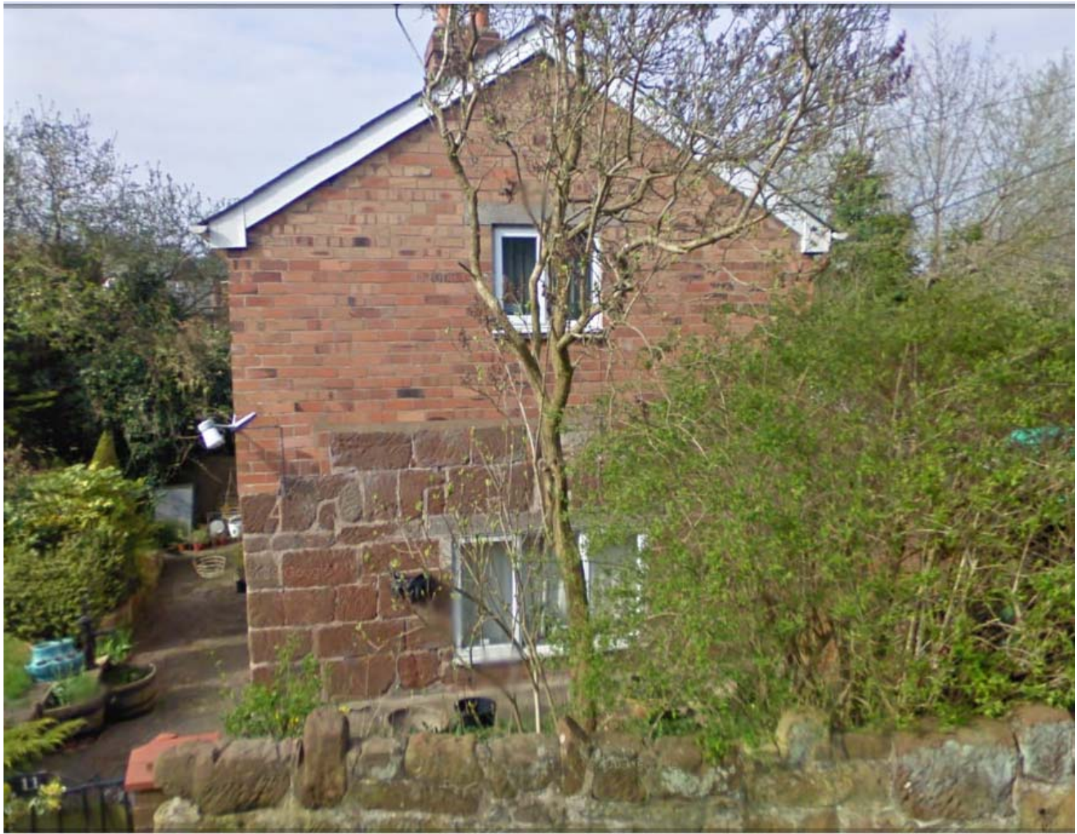
Some of the old cottages show signs of additions No.11 Brookside
