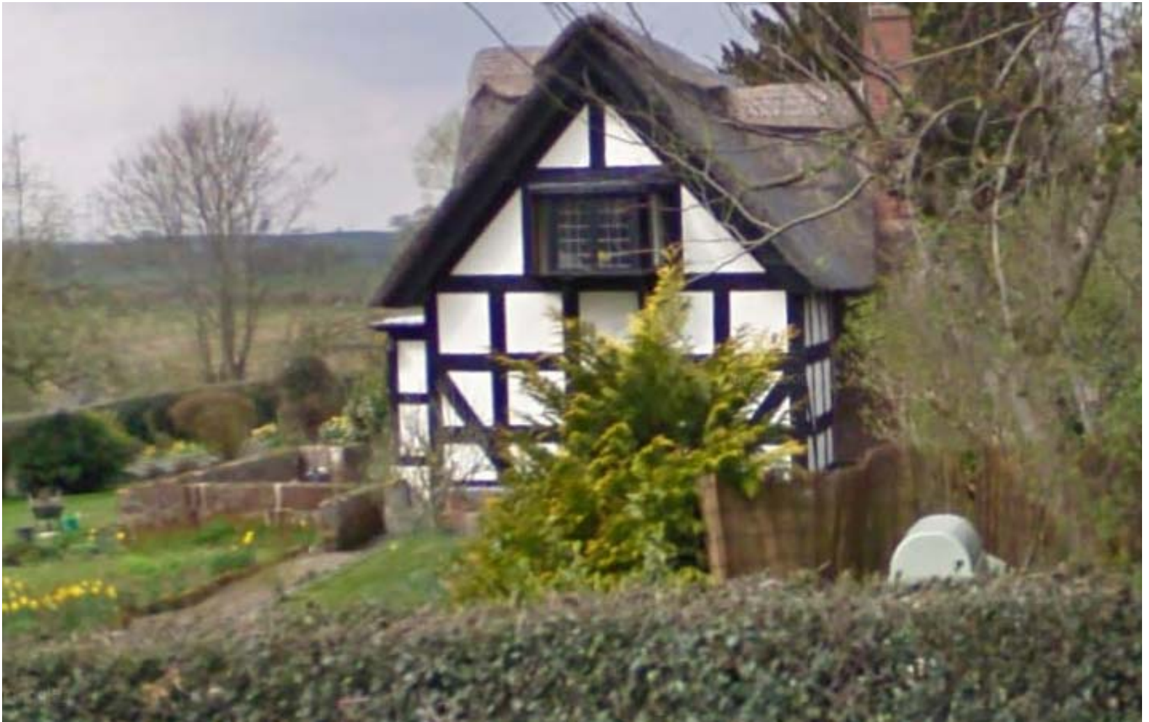
Tan House side view
